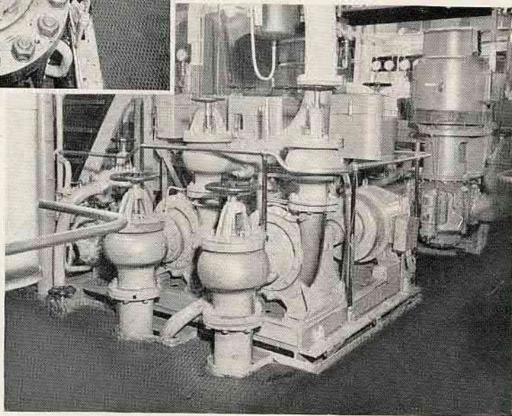
View of fuel transfer pumps and a fuel purifier (below) and the Diesel and lubricating oil centrifuges (right).
